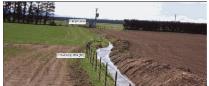
Effects of fault rupture on previously straight fence and water race. (See / voir page 195.)
